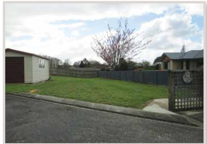
STORMWATER DRAIN UPGRADE - ST ANDREW'S COURT TE KUITI (2012/13)
