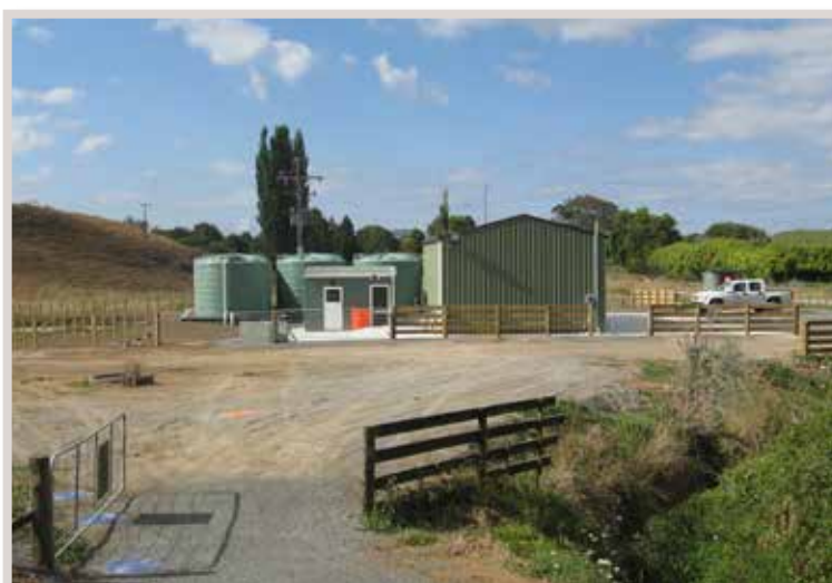
PIOPIO WATER TREATMENT PLANT
